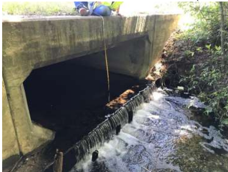
PLATE I – FIELD REVIEW OF NORMAL WATER LEVEL (NWL) AT THE 10'x3' CBC CROSS DRAIN AT STA 778+00 IN BASIN B (4/6/2017)
